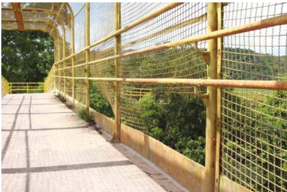
Photographs 81: Overpass located in Vila Concórdia. Overpass' protective mesh in precarious conditions.
